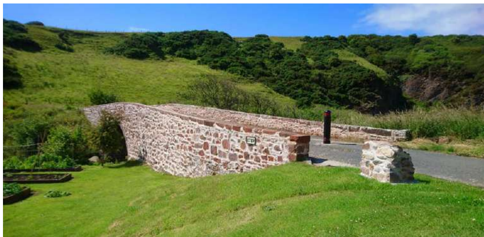
The new Cairn at Nethermill Bridge.
