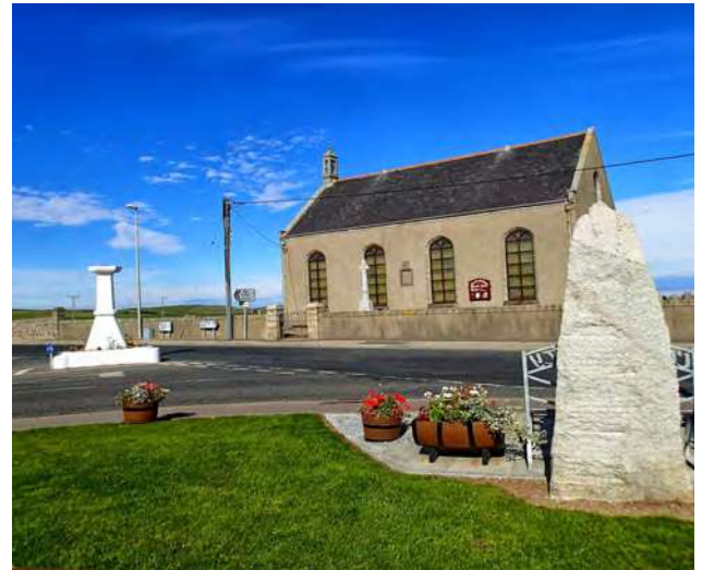
New Aberdour Parish Hall
